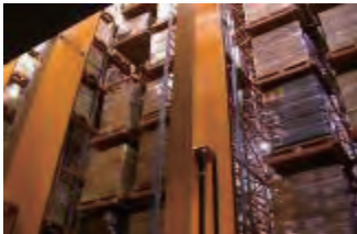
Automated Storage / Retrieval System
