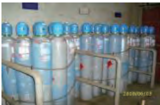
Special Gas Cylinder Warehousing
