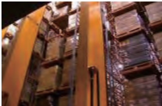
Automated Storage / Retrieval System
